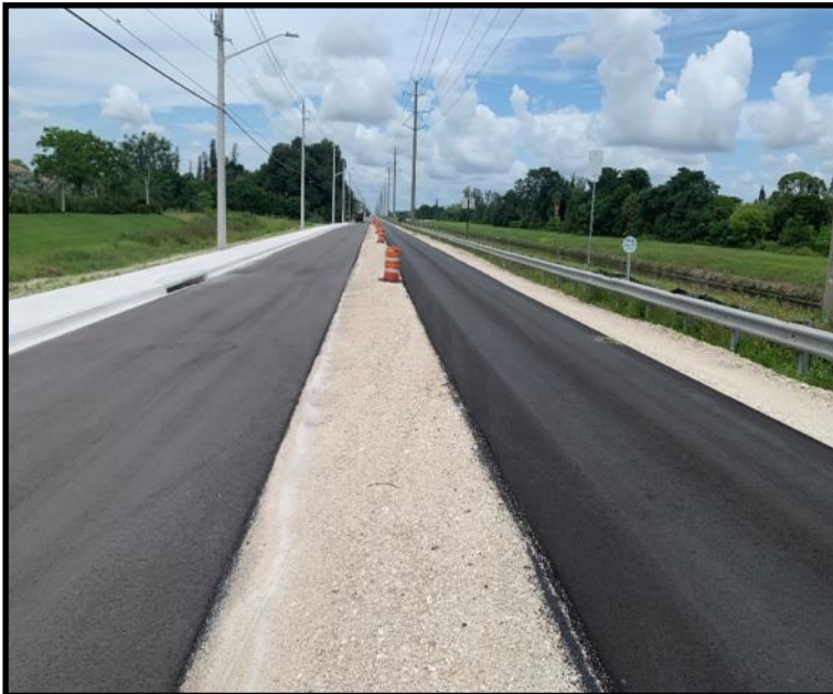
Asphalt placement
