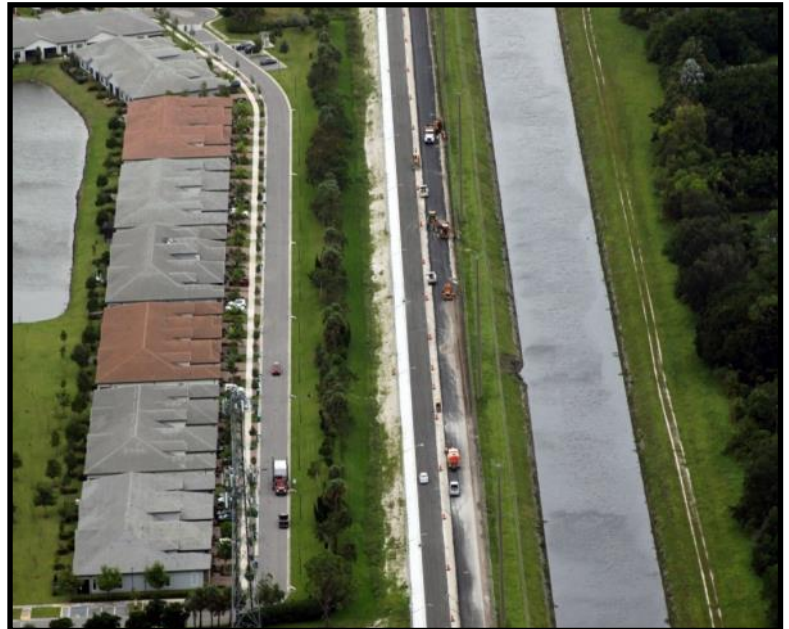
Removal of existing guardrail
